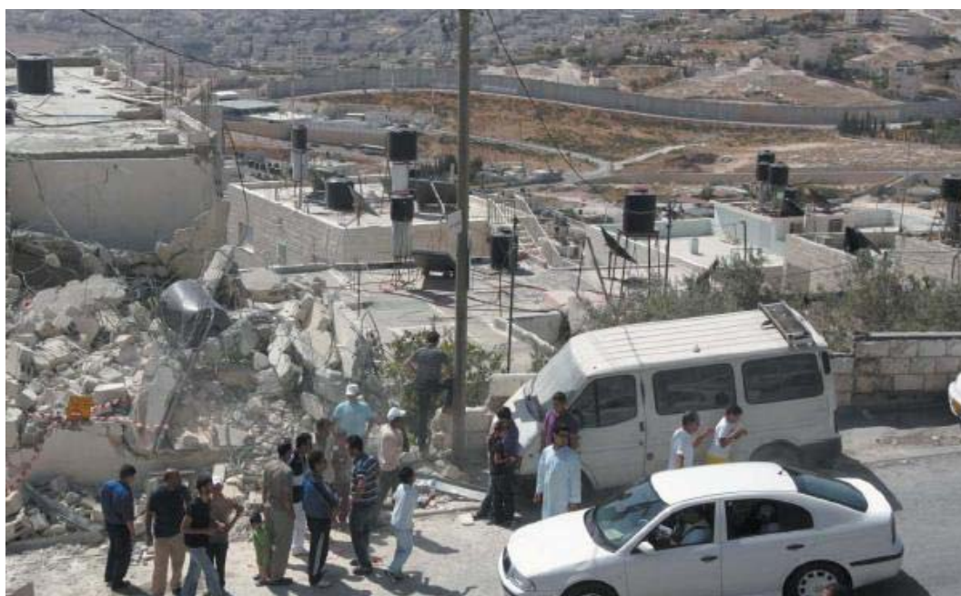
Khaled Abu Joma's house, which was demolished by Israeli Occupation Forces in Jerusalem on 30 June 2009
