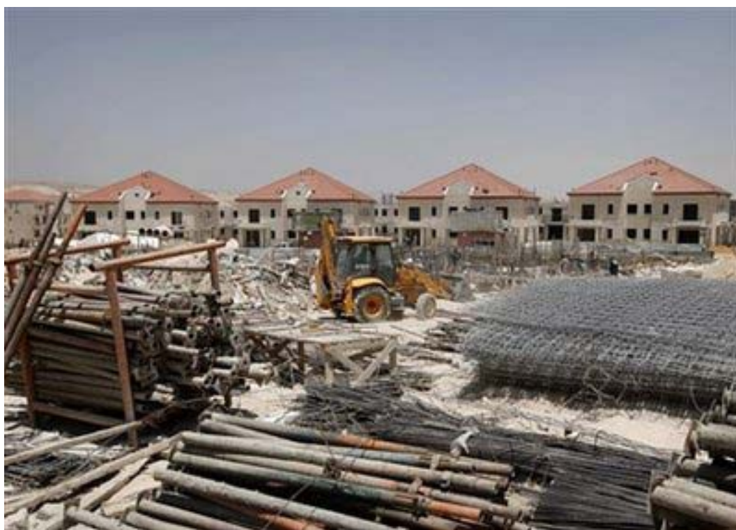
Continued construction in "Ma'ale Adomim" settlement near occupied Jerusalem
